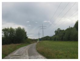
FIGURE 24.9 This high-voltage traction power line running to Eutingen Railway Substation in Germany radiates electromagnetic waves with very long wavelengths. (credit: Zonk43, Wikimedia Commons)
