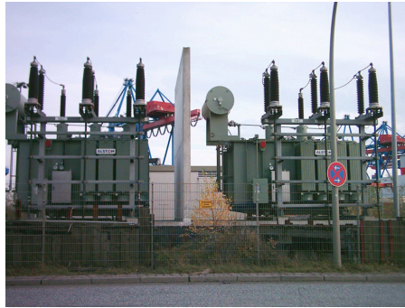
FIGURE 20.17 Power is distributed over large distances at high voltage to reduce power loss in the transmission lines. The voltages generated at the power plant are stepped up by passive devices called transformers (see Transformers ) to 330,000 volts (or more in some places worldwide). At the point of use, the transformers reduce the voltage transmitted for safe residential and commercial use. (Credit: GeorgHH, Wikimedia Commons)
