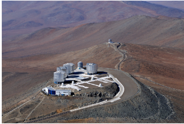
Figure 6.12 High and Dry Site. Cerro Paranal, a mountain summit 2.7 kilometers above sea level in Chile's Atacama Desert, is the site of the European Southern Observatory's Very Large Telescope. This photograph shows the four 8-meter telescope buildings on the site and vividly illustrates that astronomers prefer high, dry sites for their instruments. The 4.1-meter Visible and Infrared Survey Telescope for Astronomy (VISTA) can be seen in the distance on the next mountain peak. (credit: ESO)
