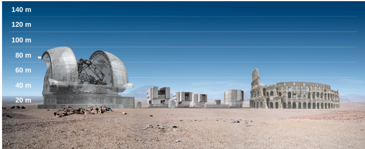
Figure 29.6 European Extremely Large Telescope, European Very Large Telescope, and the Colosseum. The European Extremely Large Telescope (E-ELT) is currently under construction in Chile. This image compares the size of the E-ELT (left) with the four 8-meter telescopes of the European Very Large Telescope (center) and with the Colosseum in Rome (right). The mirror of the E-ELT will be 39 meters in diameter. Astronomers are building a new generation of giant telescopes in order to observe very distant galaxies and understand what they were like when they were newly formed and the universe was young. (credit: modification of work by ESO)
